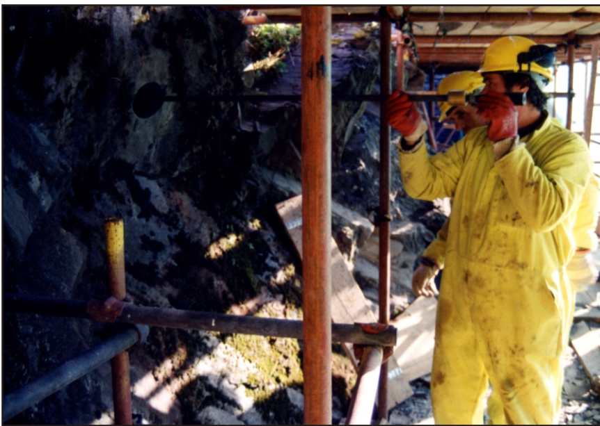
Fibregrip® Rockbolt being inserted into a 32mm diameter hole containing two 800mm long resin capsules.
