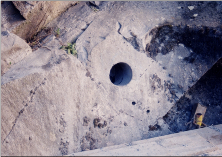
Rotary percussive drilled holes, over cored to a depth of 250mm.
