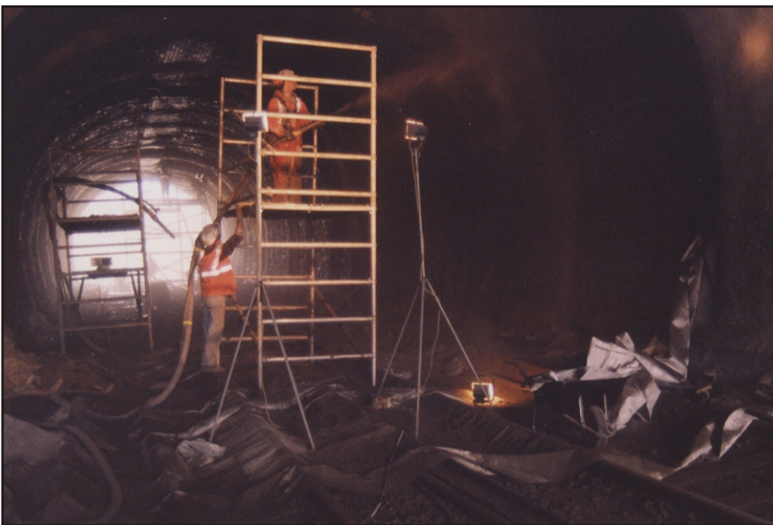
Shotcreting a 150mm thick permanent arch between toe blocks.
