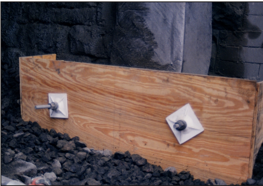
Toe block cast around Fibregrip® Rockbolts.
