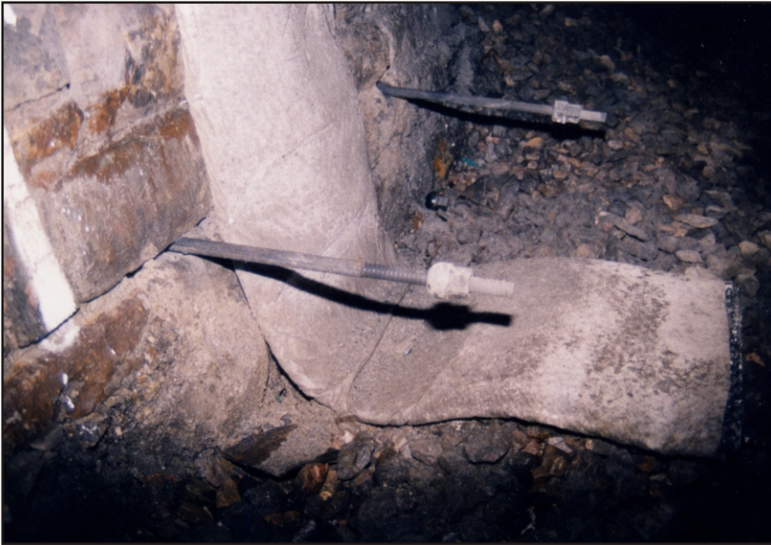
Fibregrip® Rockbolts installed at 750mm centres to secure the toe blocks.
