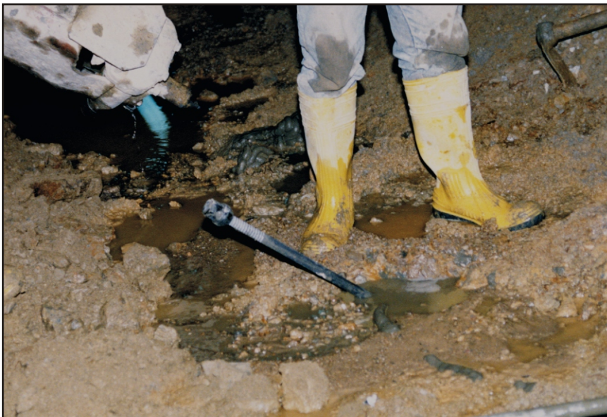
Installed floor bolt
