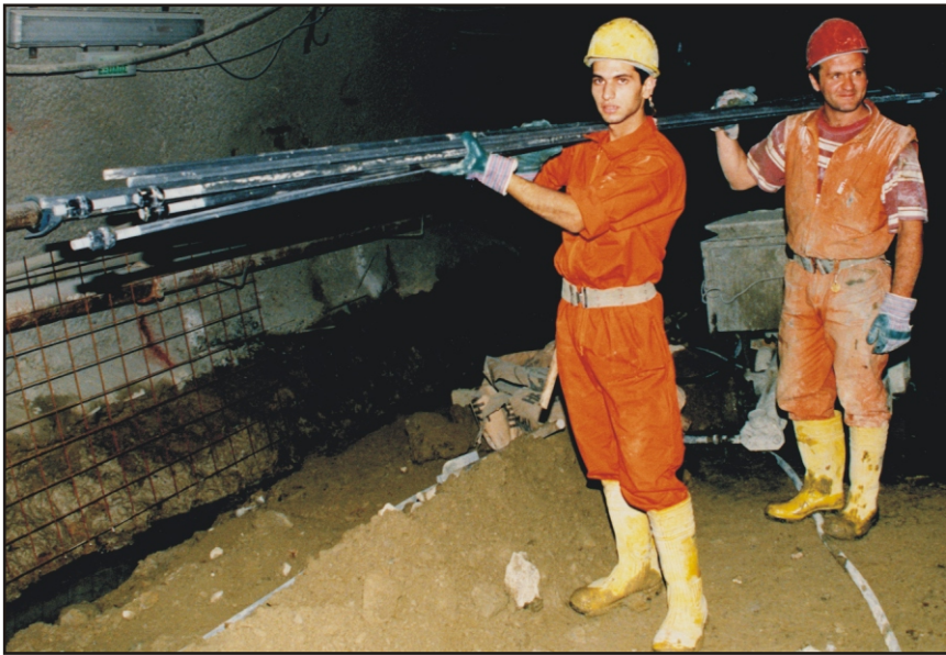
Lightweight Fibregrip® bolts gave better handleability
