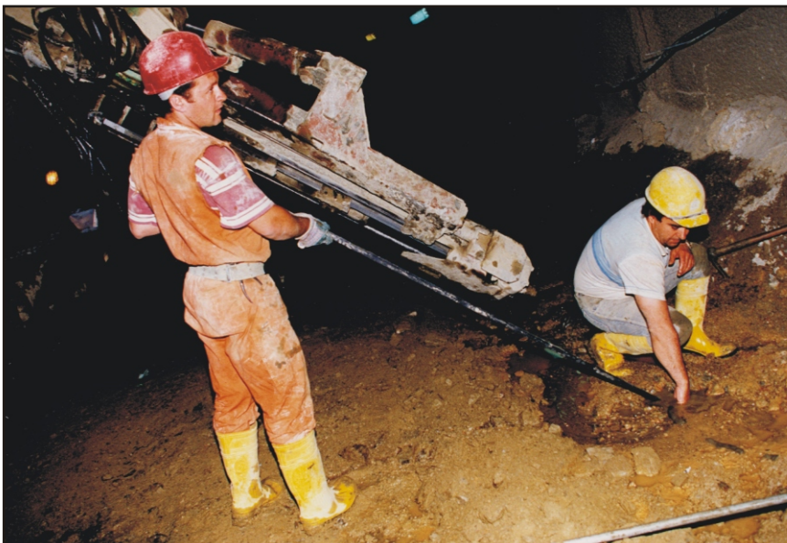
Installing rockbolts into floor
